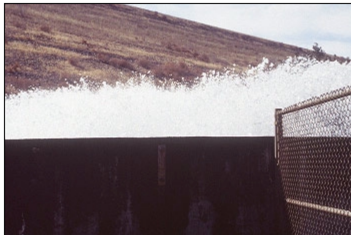
Aerator at the Mokelumne Hatchery
